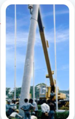
by Lifting Crane
