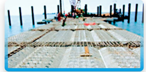
PRECAST HALF SLAB
