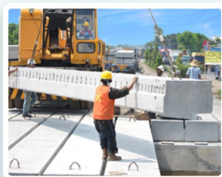
PC Voids Slab or PC Chanel Girder
