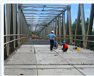
Double Tee Slab for Truss Bridge
