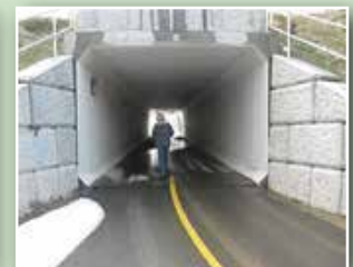
Pedestrian Crossing Underpass
