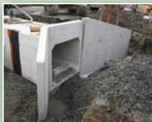
Box Culvert Installation
