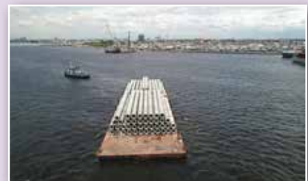
Cylinder Pile Distribution
