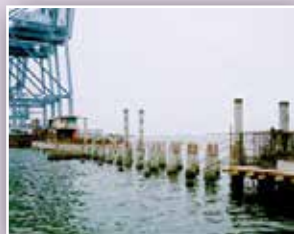
Piles for Marine Structures
