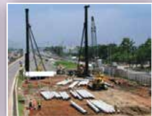
Piles Foundation for Bridges
