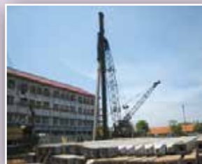
Piles Foundation for Building
